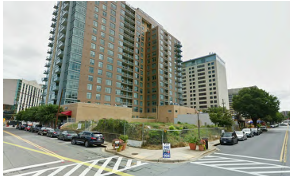
2. CORNER OF AUBURN AVE AND NORFOLK AVE
